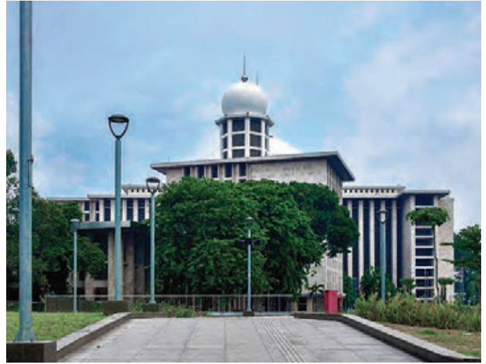
A 45m-diameter central spherical dome covers the main prayer hall
